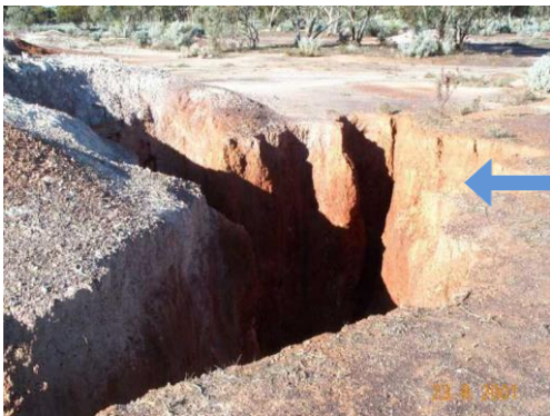
Active mine shaft
